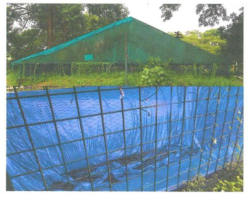
Fig 2.5 One lakh litre tank for rainwater harvesting
